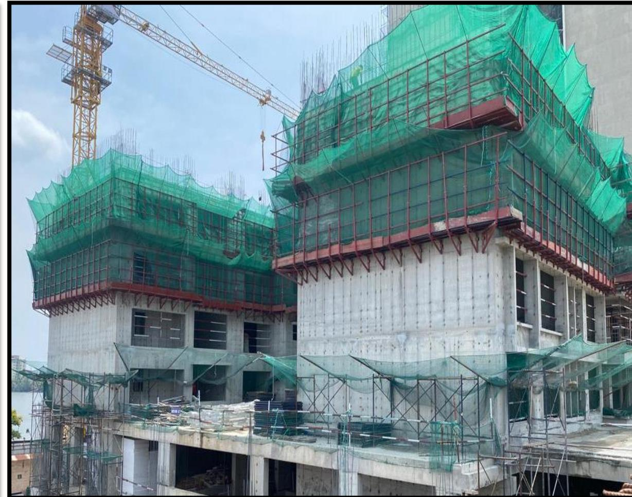
**Third floor roof slab casted. Fourth floor roof slab pour 1 reinforcement in progress**
