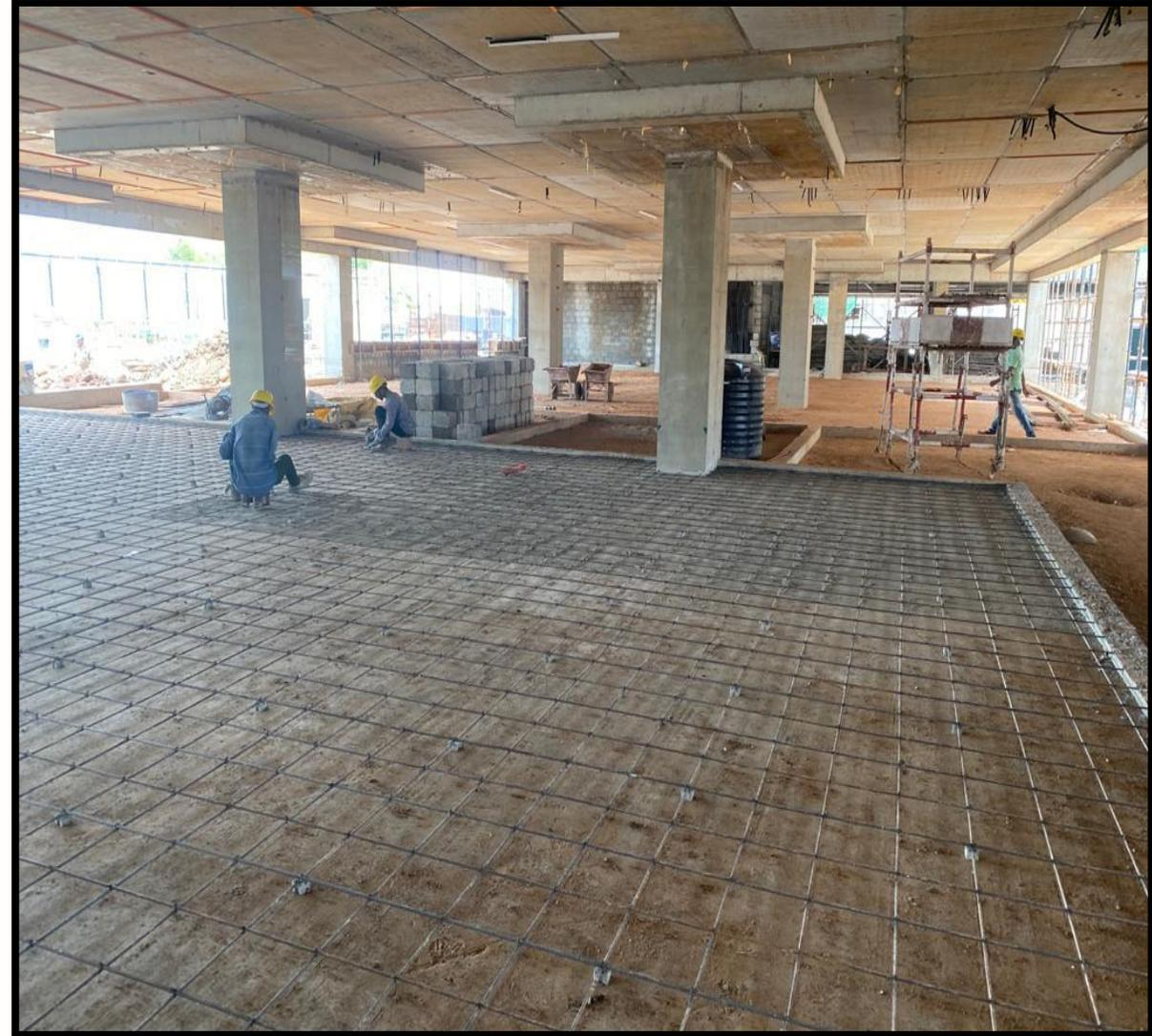
**Backfilling completed. Grade slab works in progress**
