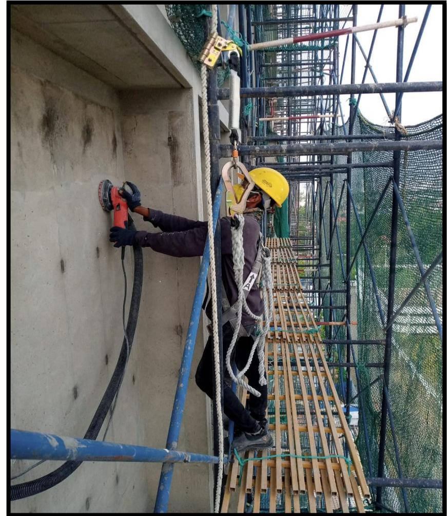
**External grinding works in progress**
