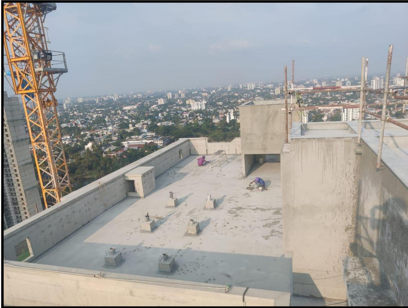
**Structure completed. Terrace waterproofing & protective screed 2/4 flats completed**
