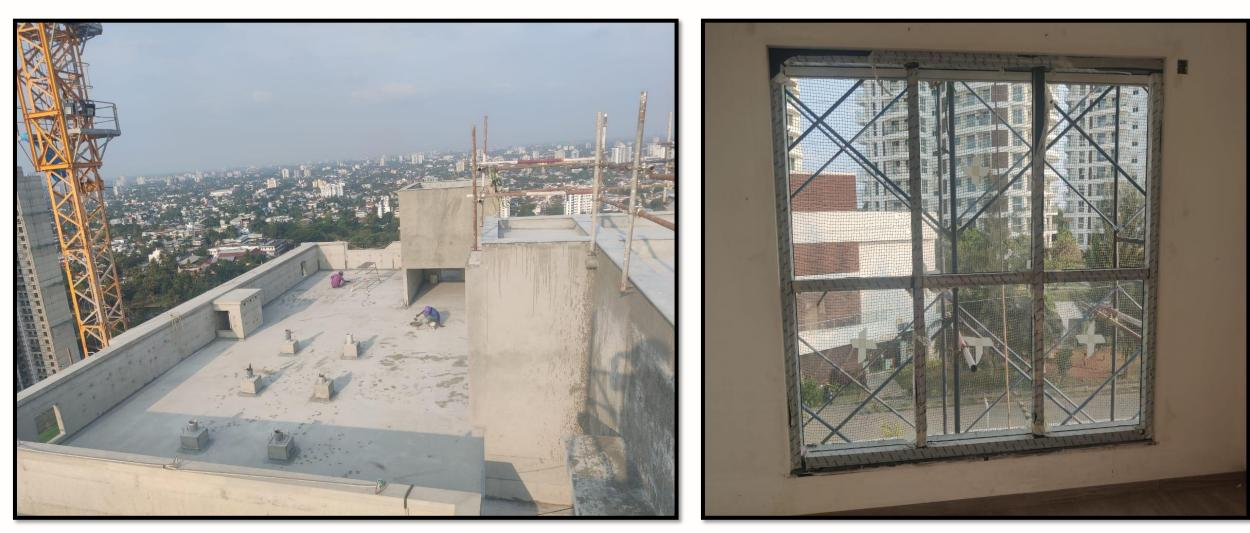
Structure completed. Terrace waterproofing & protective screed 2/4 flats completed SGML works 10 floors in progress
