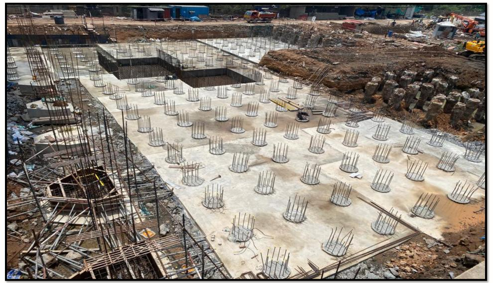
Excavation 100% completed. Pile chipping 100% completed. PCC 100% completed. Raft steel works in progress.
