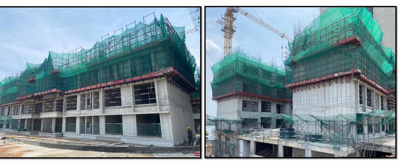
Third floor roof slab casted. Fourth floor roof slab pour 1 reinforcement in progress
